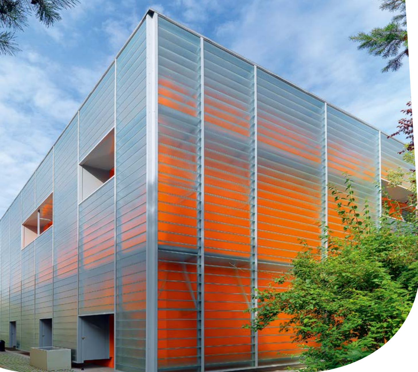
TECHNOPOLIS, Wrocław, Poland
