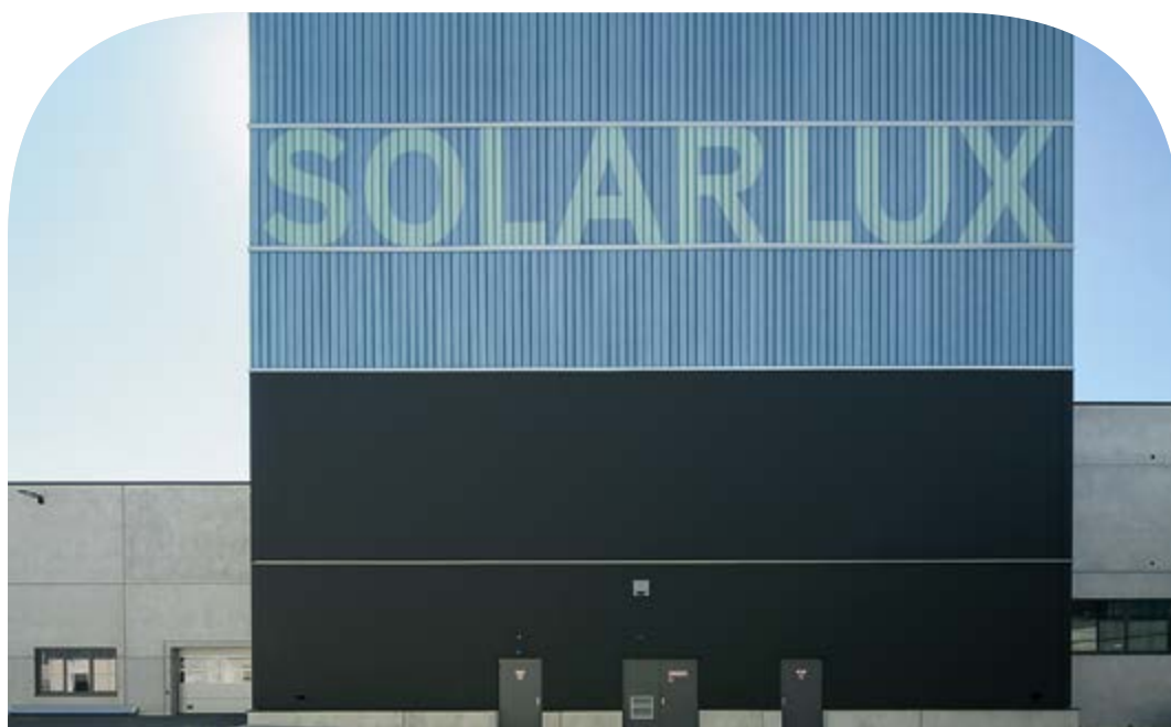
SOLARLUX Campus, Melle, Germany
